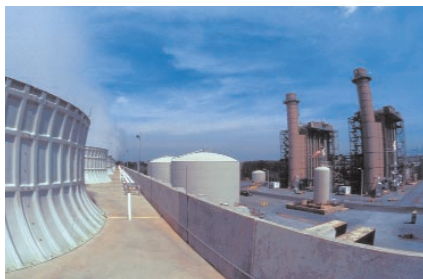
AEC's generating facilities are built with state-of-the-art generating equipment.
