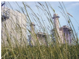
The James A. Vann, Jr. Combined-Cycle Power Plant uses the most cost-efficient forms of electric generation capacity available.
