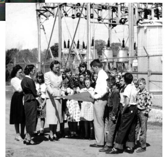
Early tours of AEC's substations educated children about transmitting electricity.
