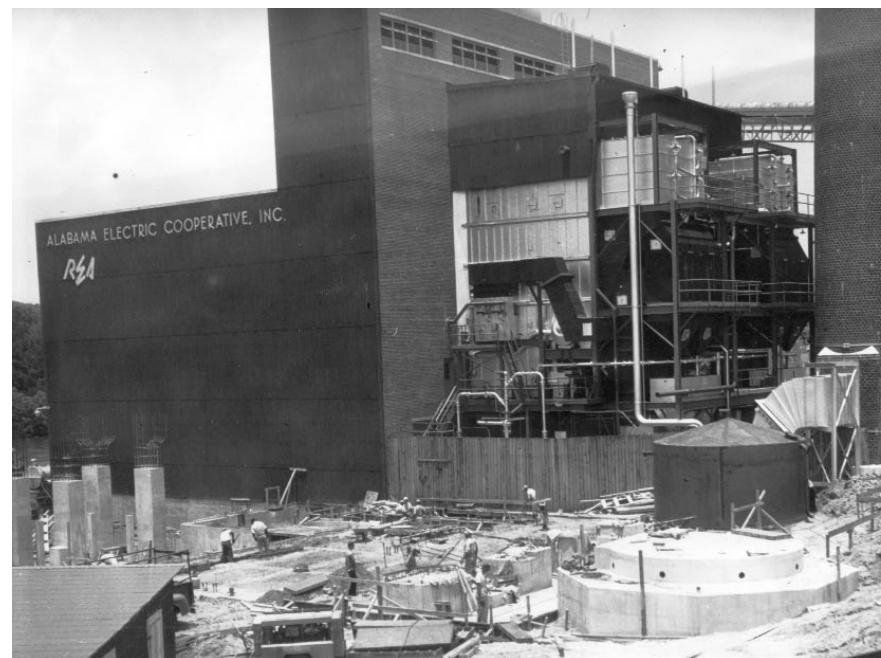
The Maury A. McWilliams Power Plant, constructed in the 1950's was AEC's first self-built generating facility.
